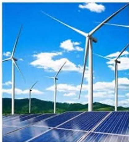
Solar power station
