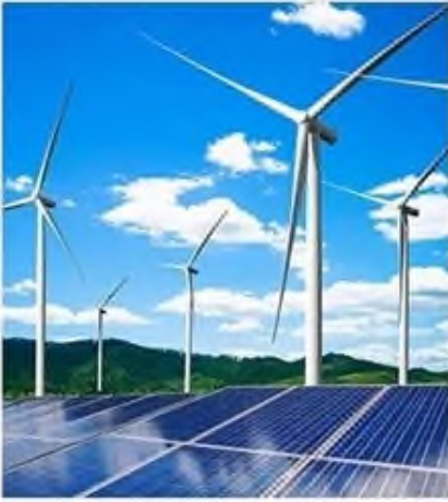
Solar power station
