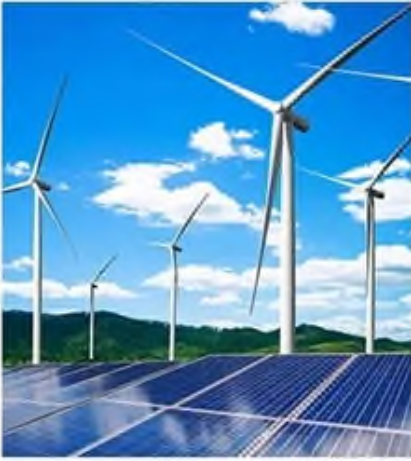
Solar power station
