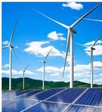
Solar power station
